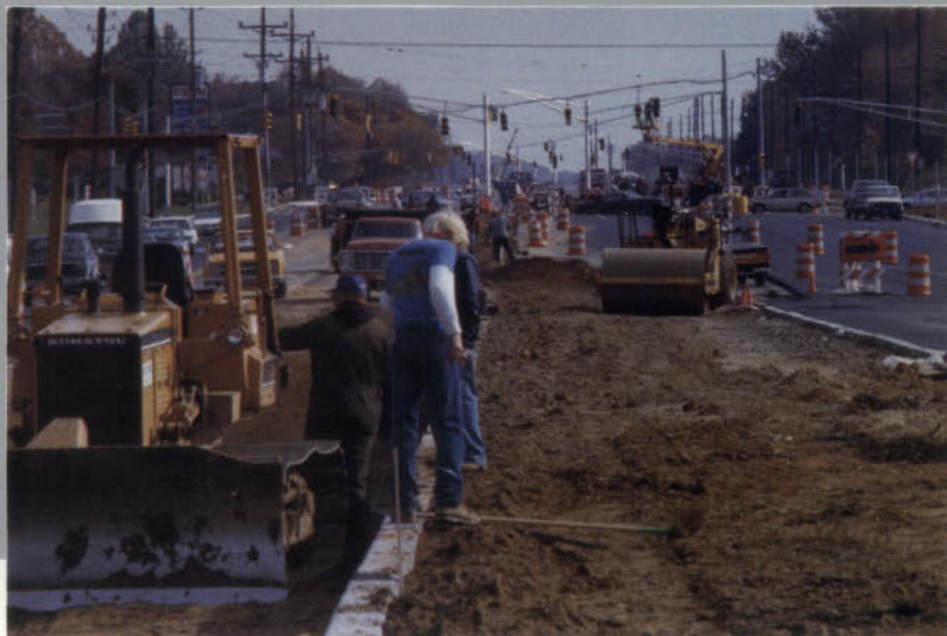
Crews work on improvements to County Route 541 in Burlington County.
