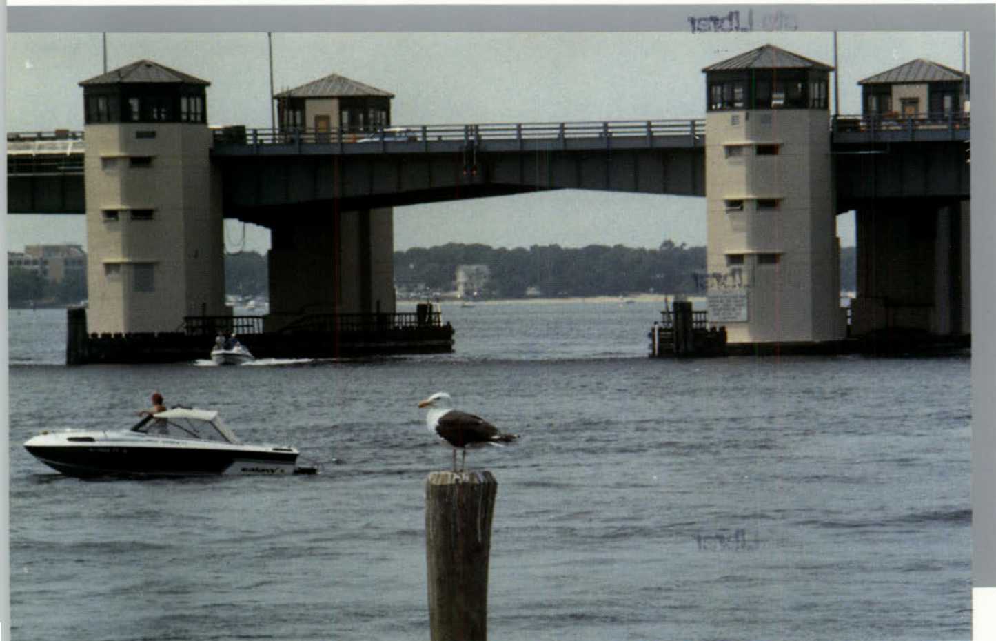
The Route 35 bridge over the Mansquan River was one of several movable bridges which received a complete overhaul this year.
