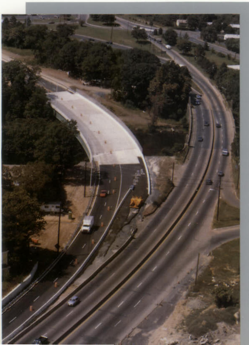
The new Route 18 bridge over the Lawrence Brook in East Brunswick opened to traffic in September.
