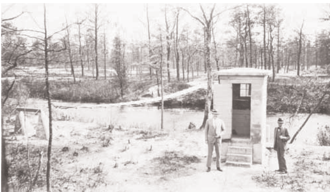
Figure 3. USGS streamflow-gauging station on the Toms River as it appeared in 1930. The Toms River is the largest stream flowing into Barnegat Bay. The station has been used to measure the flow of the river on a continuous basis for 75 years.
