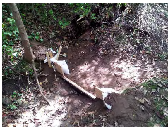
Figure 14. Weir being constructed when Brau Kettle was dry. Photo, T. Pallis.
