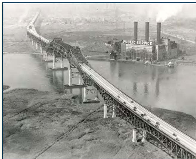
Route 1 & 9, Pulaski Skyway, between Newark and Jersey City, Essex and Hudson counties, date unknown.
