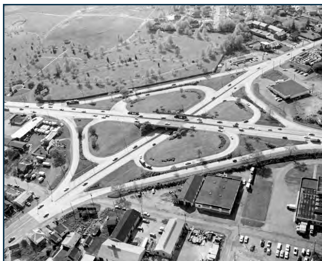
Route 1, 9, and 35 cloverleaf interchange, Woodbridge, Middlesex County, 1967.
