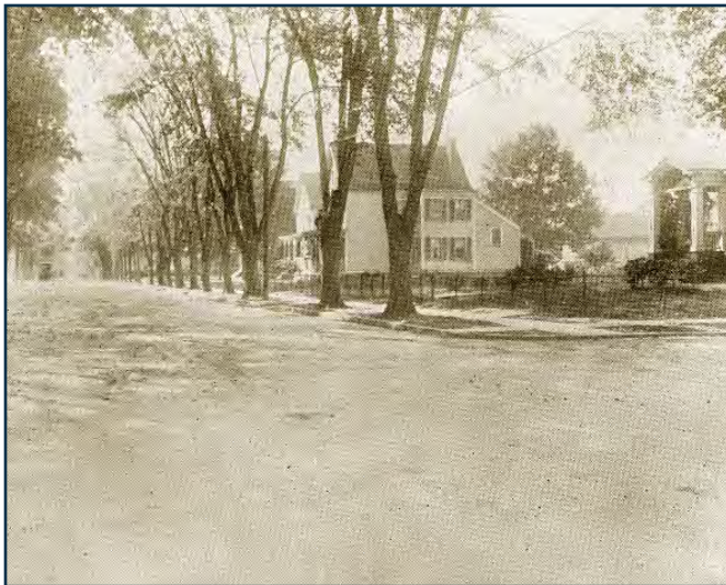
“Before” and “After” images of improvements to Chestnut Street, south of Clay Avenue, in Roselle Park, Union County, date unknown.
