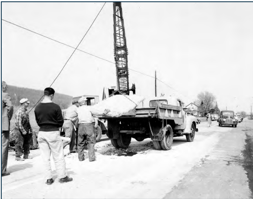
Repairs along the first concrete road in New Jersey, 1954.
