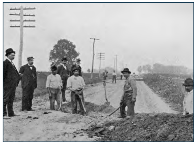
Installing under-draining system under Old York Road, Mercer County, date unknown.
