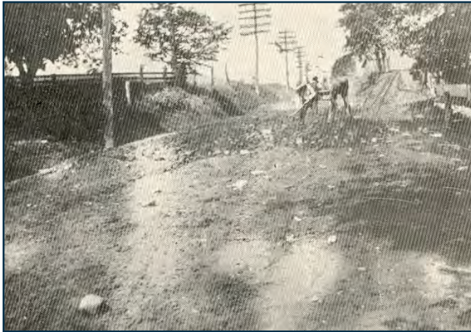
Morris Turnpike, Lopatcong Township, Warren County, before improvements, date unknown.
