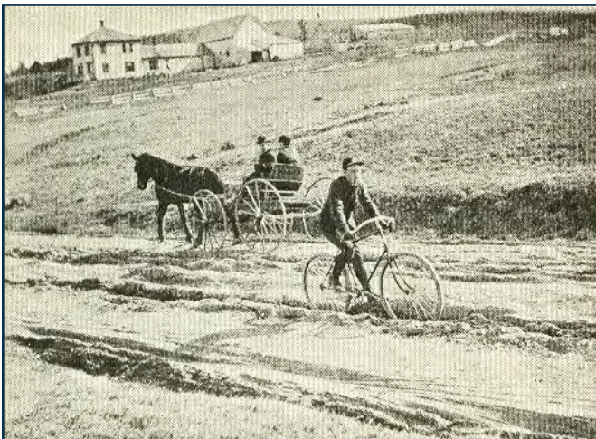
Rutting typical of undrained roadways, date unknown.
