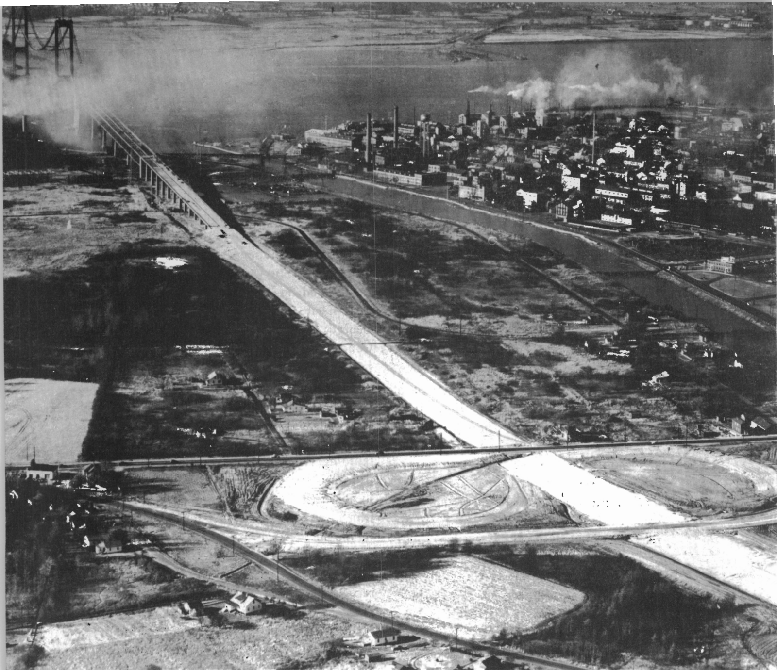
Interchange and Turnpike grading in Salem County, Delaware Memorial Bridge in background
