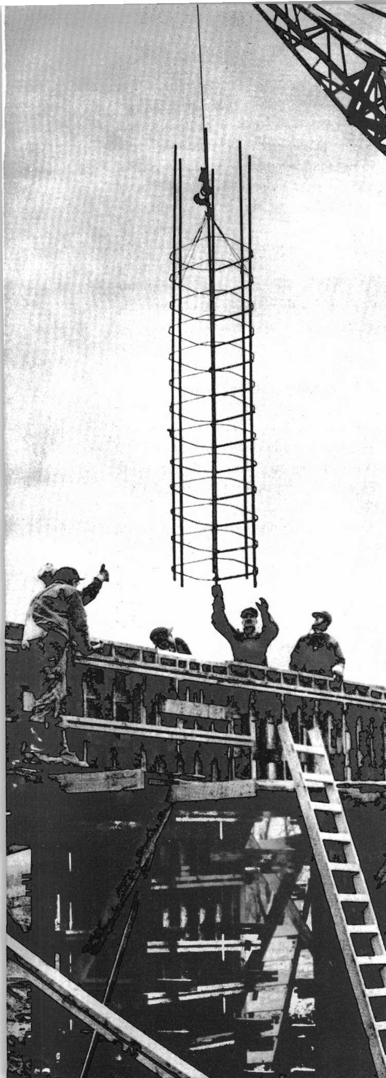
Reinforcing Steel Being Placed in Pier Forms for Swedesboro—Mullica Hill Overpass, Gloucester County
