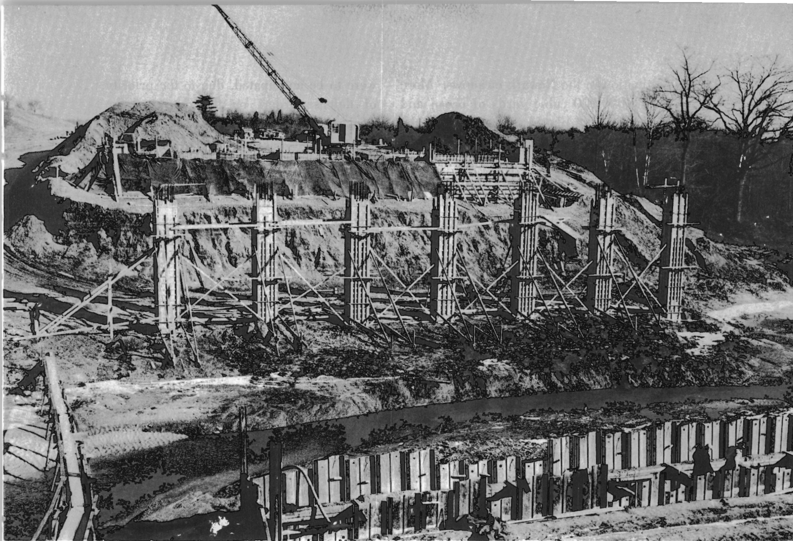
Pier Forms for Laurence Brook Overpass, Middlesex County
