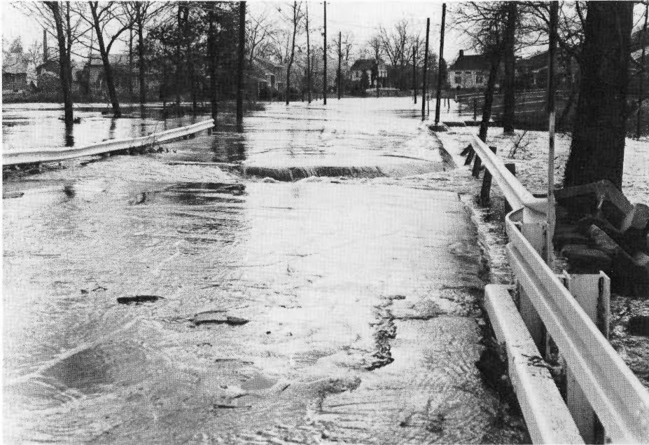
Green Brook bridge washed away
