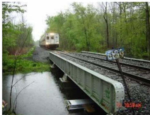
Figure 7. Three simple spans bridge used in the field tests (11)
