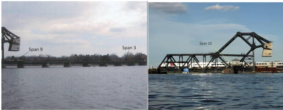
Figure 19. General view of Span 3, Span 9 and Span 12 of the Bergen County Line MP 5.48 (HX Draw) Bridge over Hackensack River Bridge from Inspection Report Cycle 4 (21)
