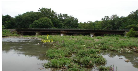
Figure 20. General view of the bridge from Inspection Report Cycle 4 (22)
