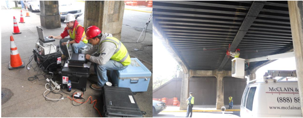
Figure 27. Sensor instrumentation and test equipment at the Main Line MP 15.95 Bridge
