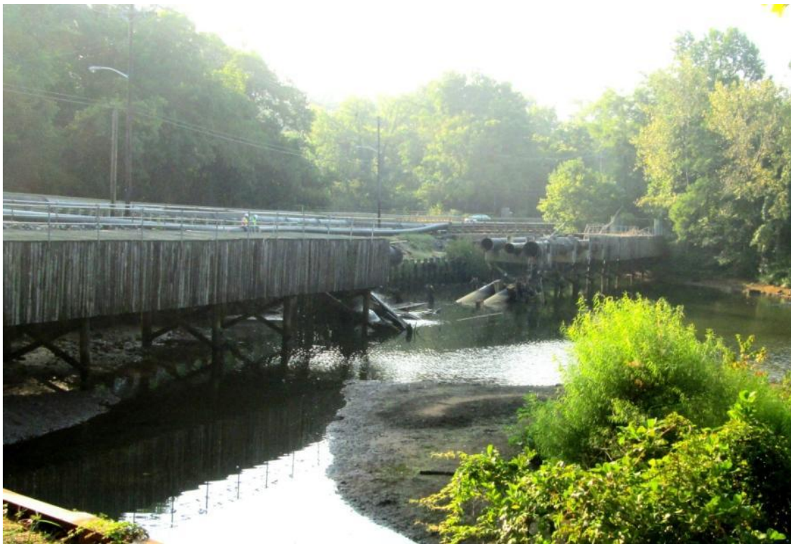
Swimming River Pipeline Bridge – August 2012. Note collapsed central portion
