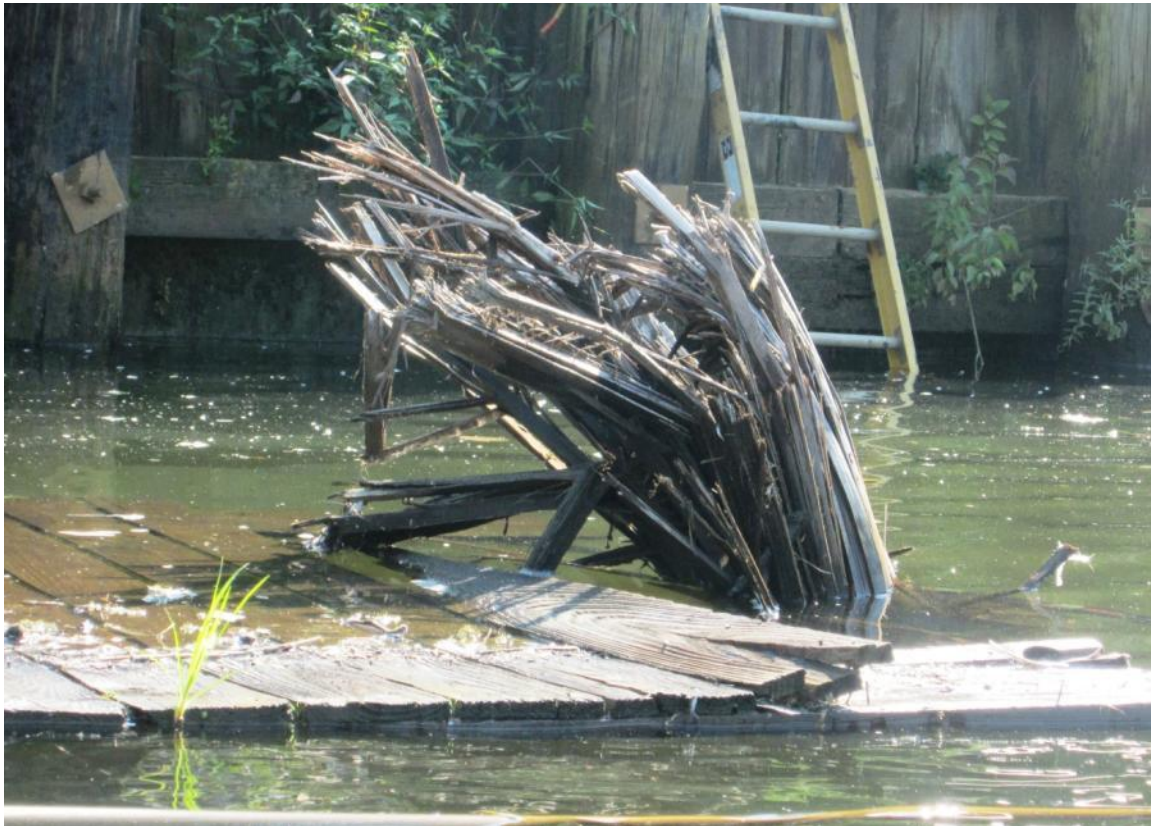
Timber Pile 5A East - Typical failed pile
