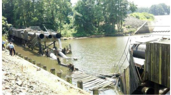
Failed Pipe Bridge
