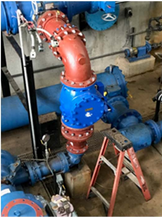
Example of one of the piping and valve replacements at the MWTP. Photo taken before painting.
