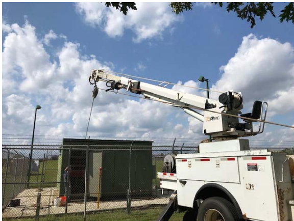
High voltage cable replacement
