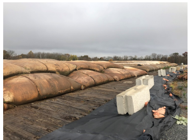
Geobags in drying (staging) area during dredging operations. Silt-laden water is directed to the geobags that filter the sediment. Clean water is discharged back to the Canal.
