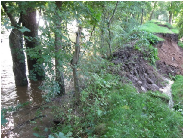
D&R Canal embankment in Stockton Borough in 2011.
