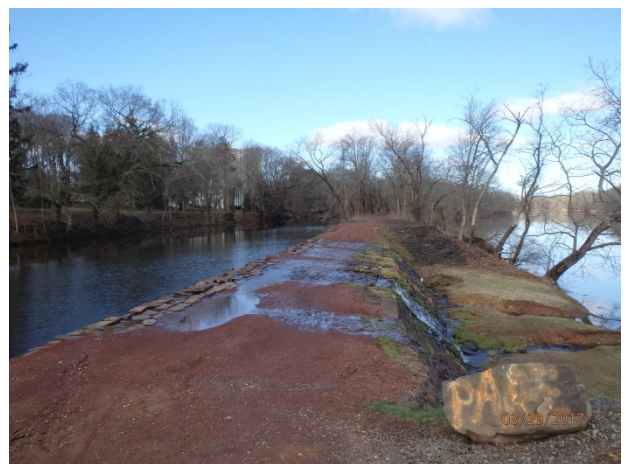
Crest of the Landing Lane Spillway.
