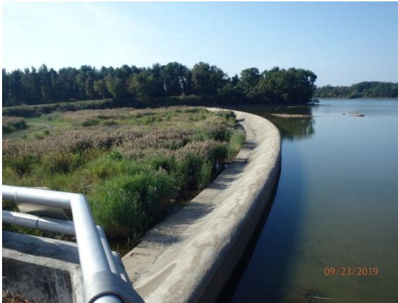
Spruce Run Reservoir Primary Spillway.
