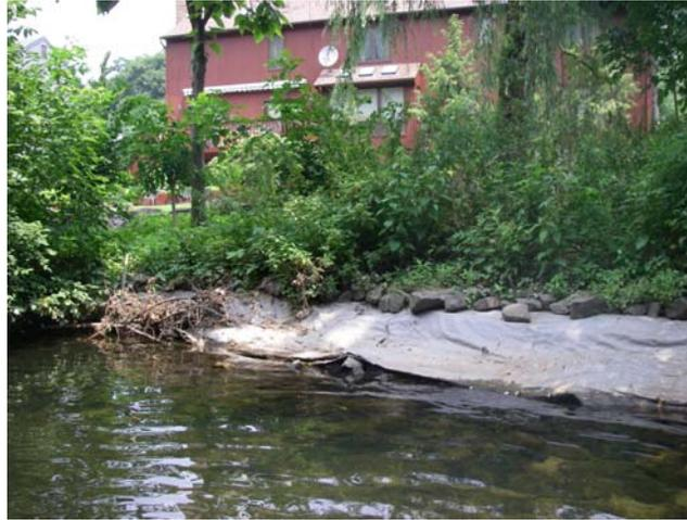
Figure 8. Fabric used to control bank erosion on Saddle River.
