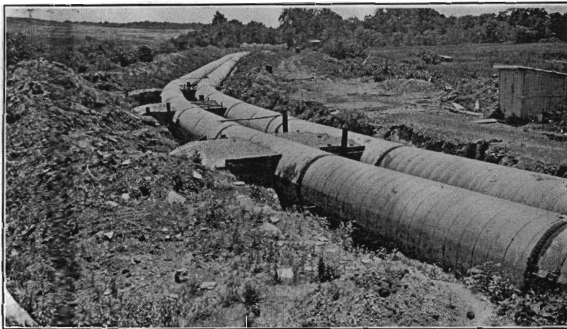
Original Wanaque Pipe Lines before covering with earth. Diameter of each is 74 inches. New line of about equal size would parallel these for three miles.
