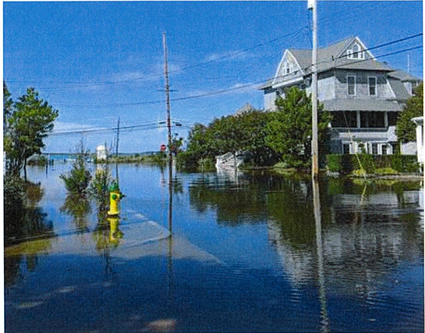
Nuisance Flooding in Seaside Park, NJ
