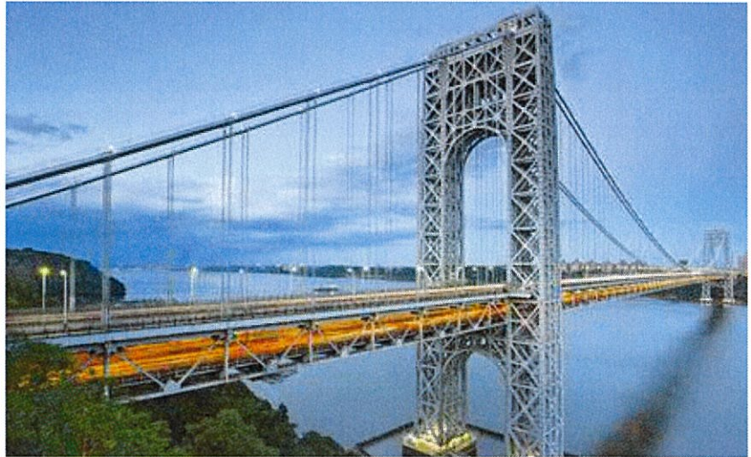
George Washington Bridge, Fort Lee, NJ
