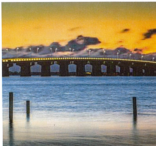
Donald J. Henderson Memorial Bridge, NJ
