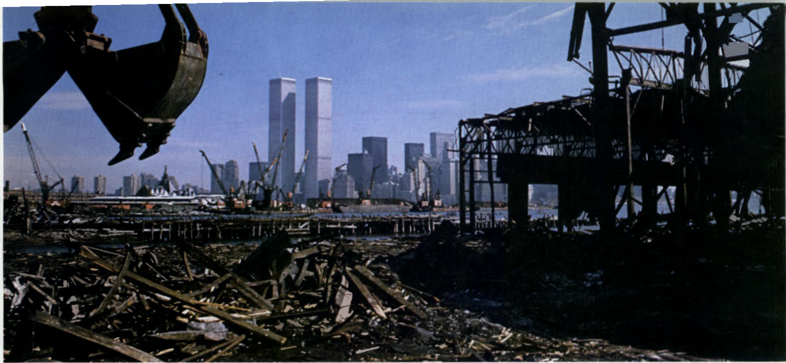
Remains of pier #14 being removed at Liberty State Park.
