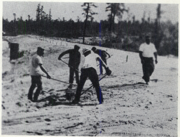
10. The final rough-grading of the dike was done with a 24-foot long railroad rail pulled by the D-8
