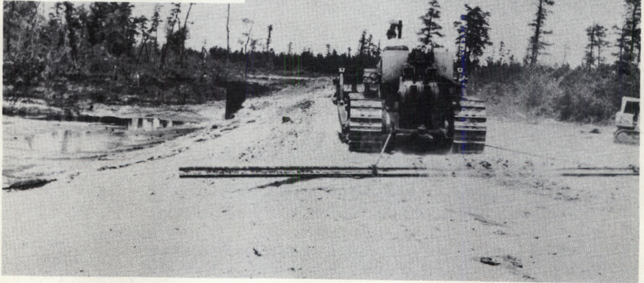
10. The final rough-grading of the dike was done with a 24-foot long railroad rail pulled by the D-8
