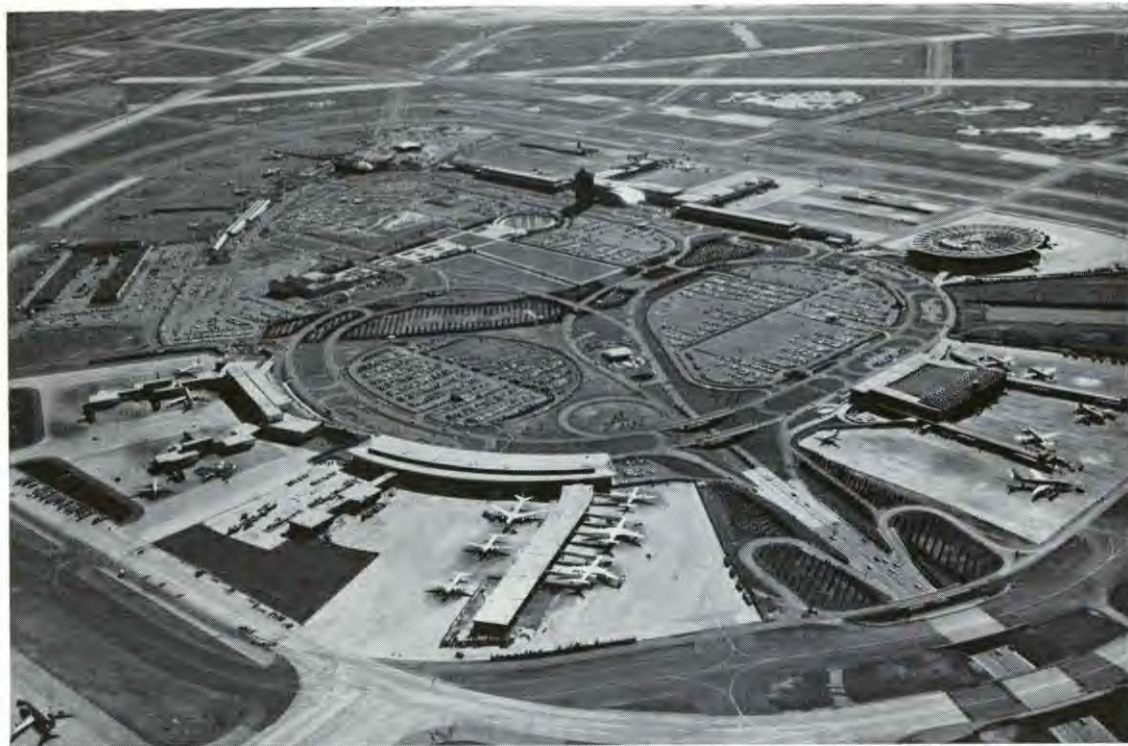
Construction of individual airline buildings in Terminal City progressed greatly with two structures completed in 1960. Work was advanced on two others, and final design work was begun on the last of the ten buildings originally planned.
