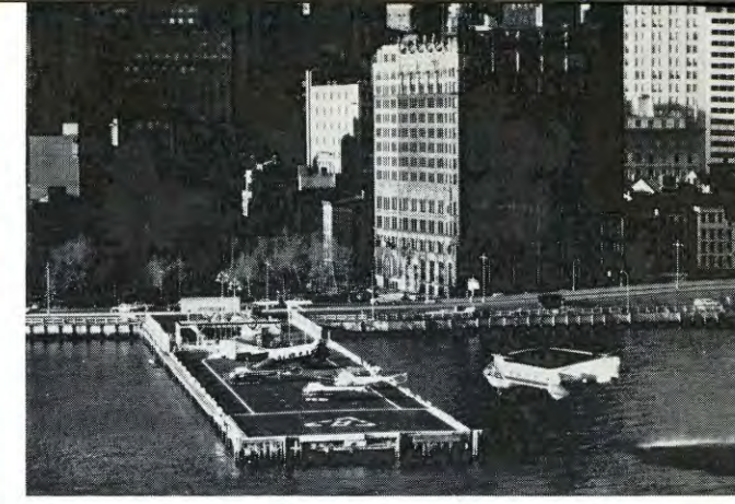
Aircraft activity at the Port Authority-Downtown Manhattan Heliport commenced on December 8, 1960. The new heliport—Manhattan's second public heliport—is located on the East River above the Battery at the foot of Coenties Slip.
