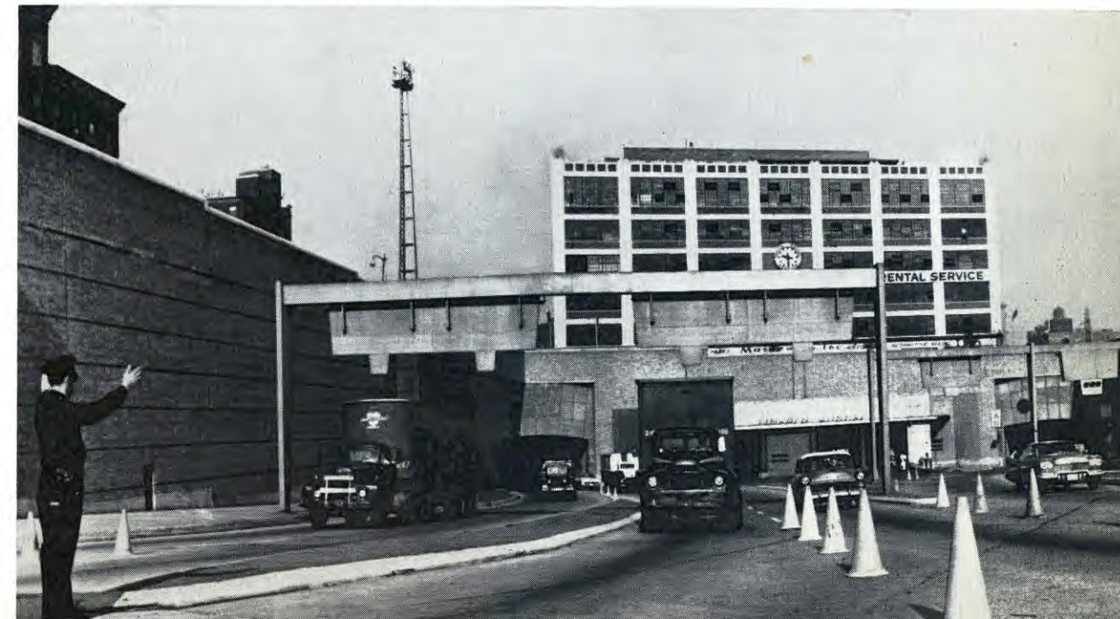
This photograph shows traffic moving on the New York exit plaza of the three-tube Lincoln Tunnel. The portal of the Third Tube, opened in May 1957, is shown on the left.
