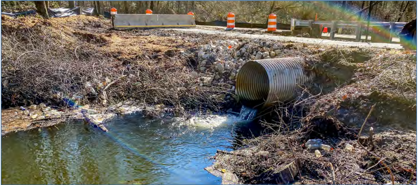
Gloucester Township: Redwood Street Culvert Replacement. SFY2024 Water Bank Long-Term Loan $1,523,477
