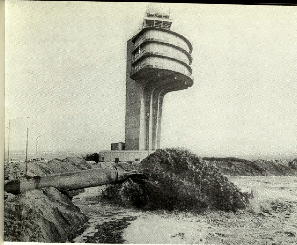
Preparation for the redevelopment of Newark Airport began in September 1964 with the start of placement of more than 12,000,000 cubic yards of hydraulic fill and surcharge over a 375 acre area in the center of the airport.
