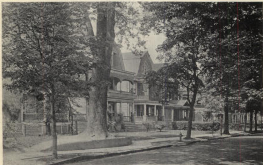
Photo by E. H. Bennett. Fig. 17: A Sidewalk Deflected and a Curb Built to Save a Fine Tree. East Orange, N. J. SHADE TREES NEED NOT ALWAYS YIELD TO STREET IMPROVEMENT.
