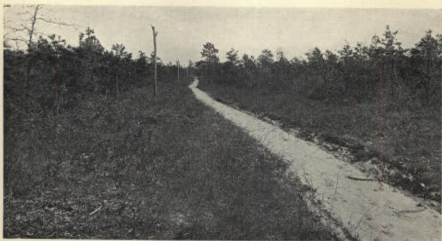
Fig. 25: Forest Fires Are Less Likely to be Started Where Roads Are Kept Clean Like This.
