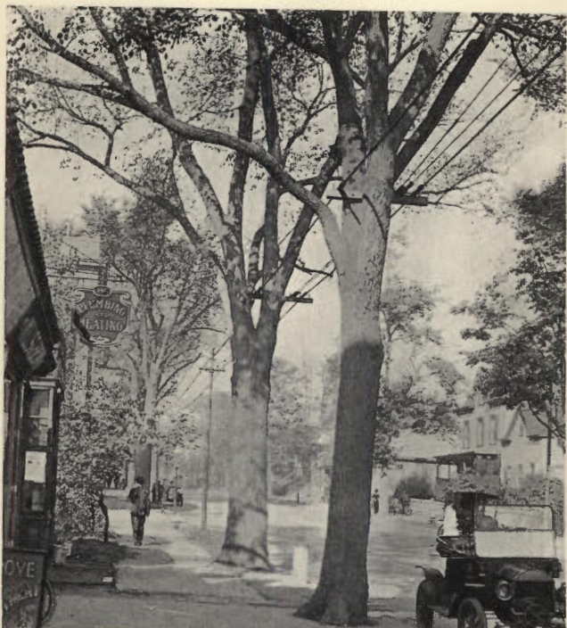
Fig. 14: A Good Way to Carry Electric Wires Through Tree Crowns. The Cross-Arms Securely Bolted to the Branches Do No Harm But Give Strength. East Orange.
