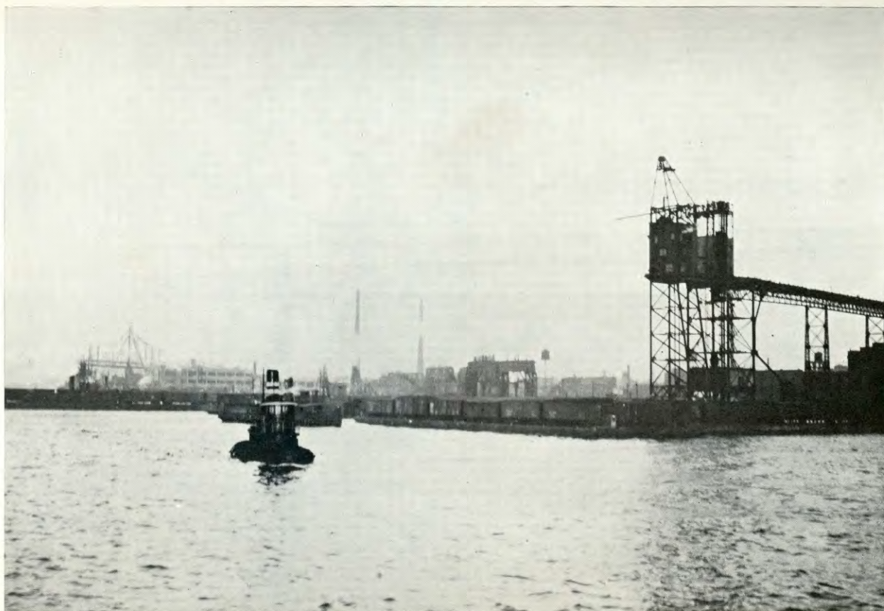
FLOATBRIDGE TERMINAL, LONG ISLAND CITY. Looking east on carfloats tied up, awaiting their turn for delivery to Long Island Railroad.
