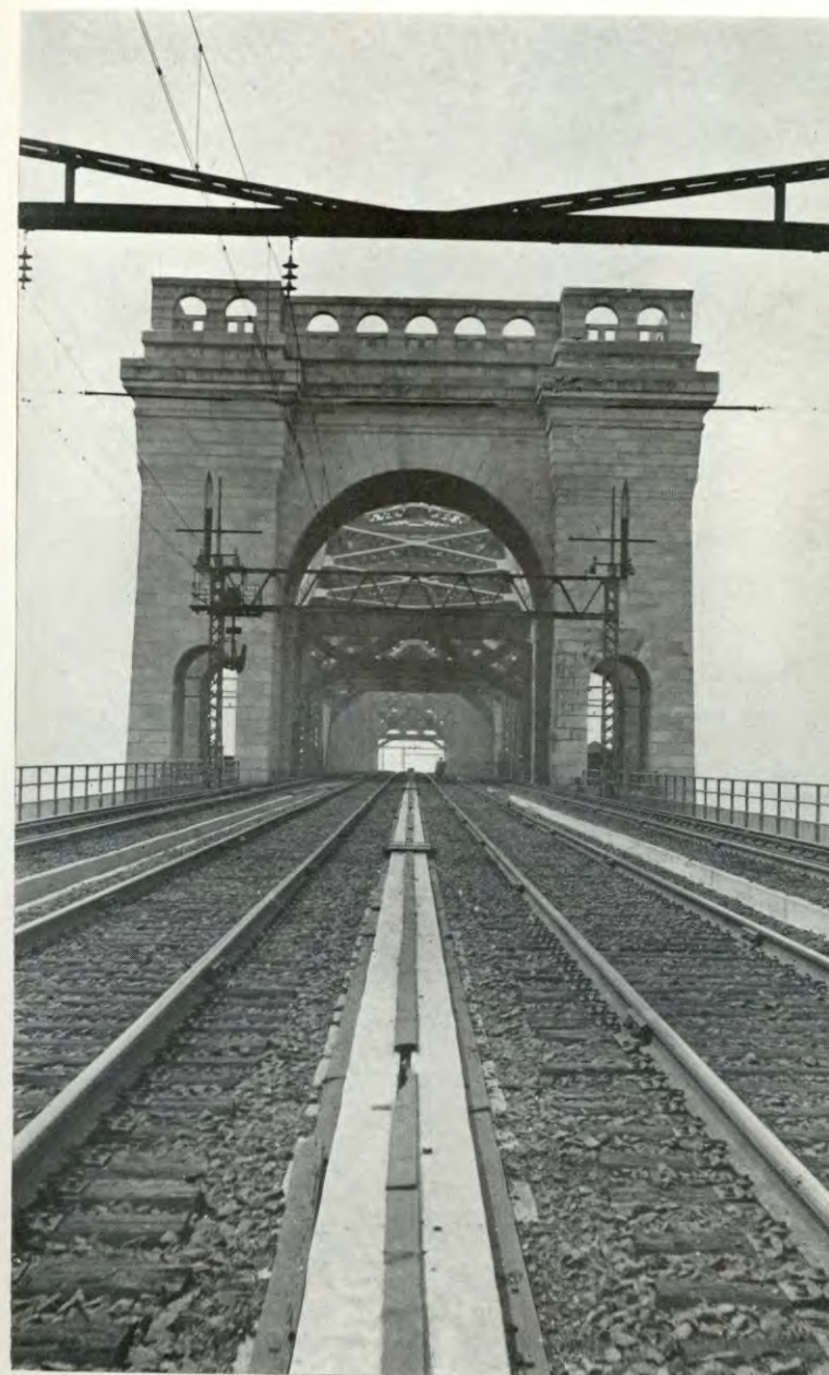
HELL GATE BRIDGE
