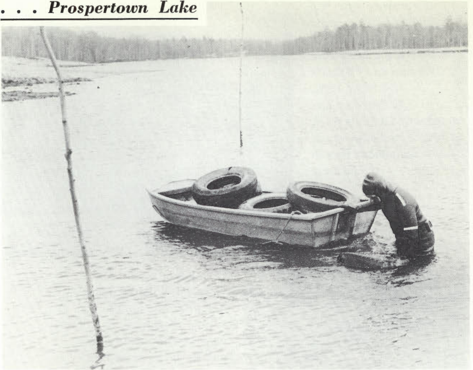
The tires were placed on the bottom of the lake in two pyramids about 20 feet in diameter
