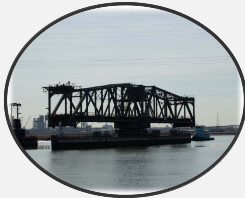
Existing Portal Bridge Structure
