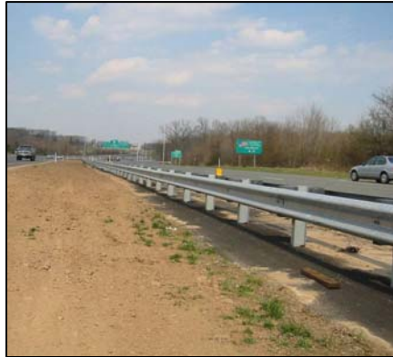
W-Beam Guide Rail Installed along Interstate 295
