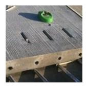
Figure 14: Rapid Roadways Barra Glide dowel system (from <u>www.rapidroadway.com/Gallery</u>).
