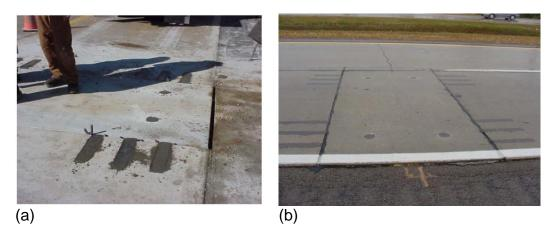
Figure 16: Michigan method precast system (a) load transfer system and grouting and (b) complete installation (Buch, 2007).
