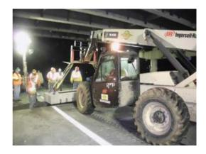
Figure 4: Fork truck installing precast panel beneath an overpass (NCPA, 2017).
