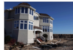
Hurricane Sandy - Shore Damage Nov. 9, 2012
