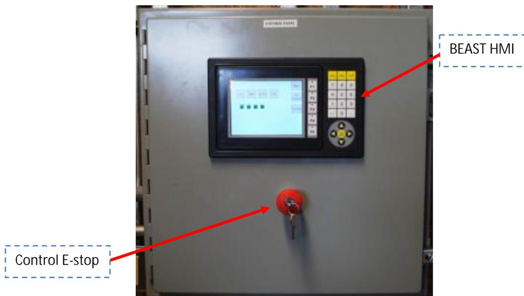
*Figure 22: Master PLC Control Box with HMI.*
