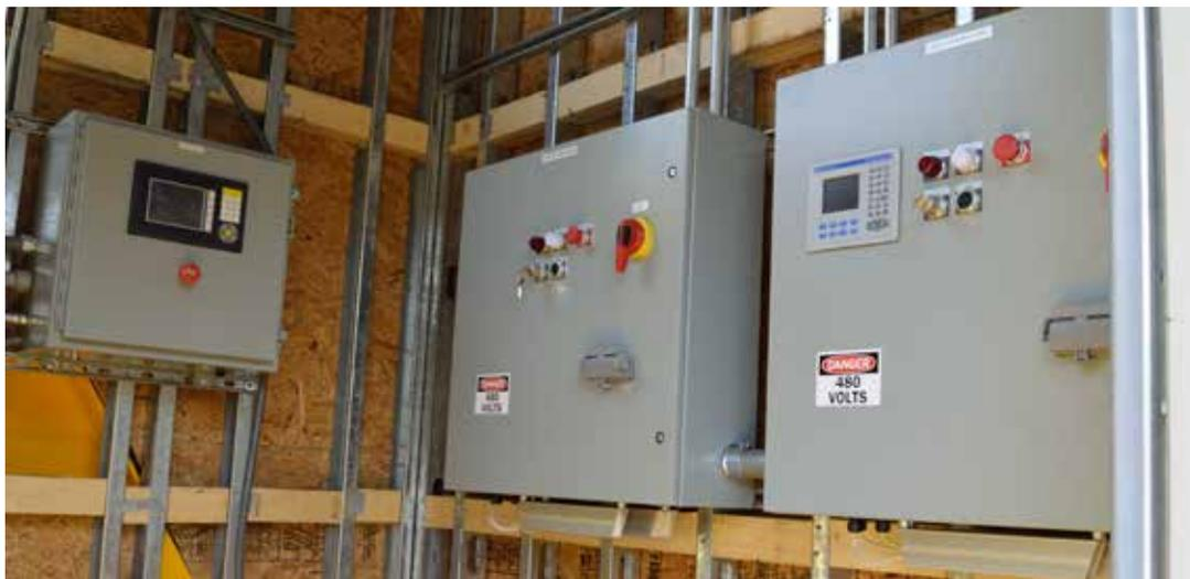
*Figure 4. Assembly Showing PLC and Rail Cart Controllers in Winch End Frame.*
