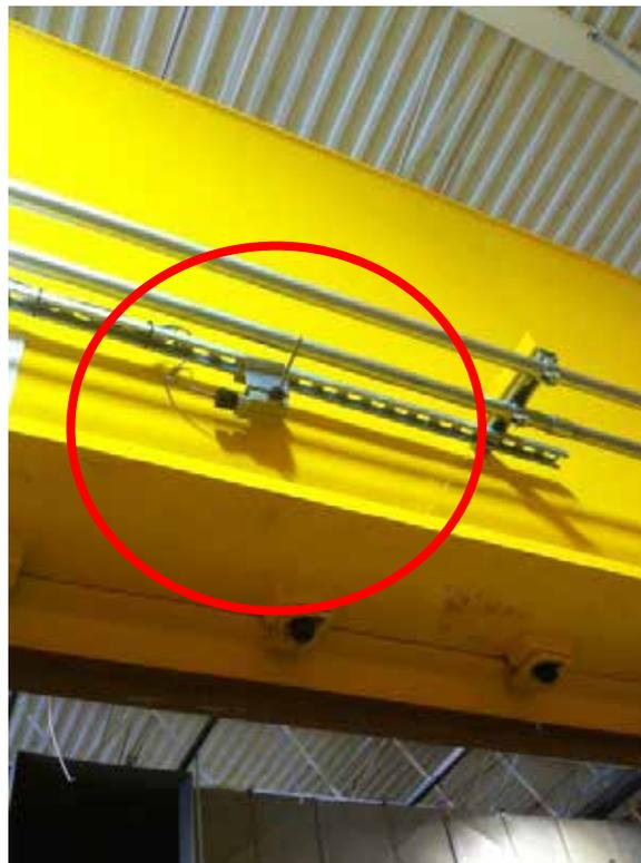
*Figure 23: Structure bumper kill switch (circled)*
