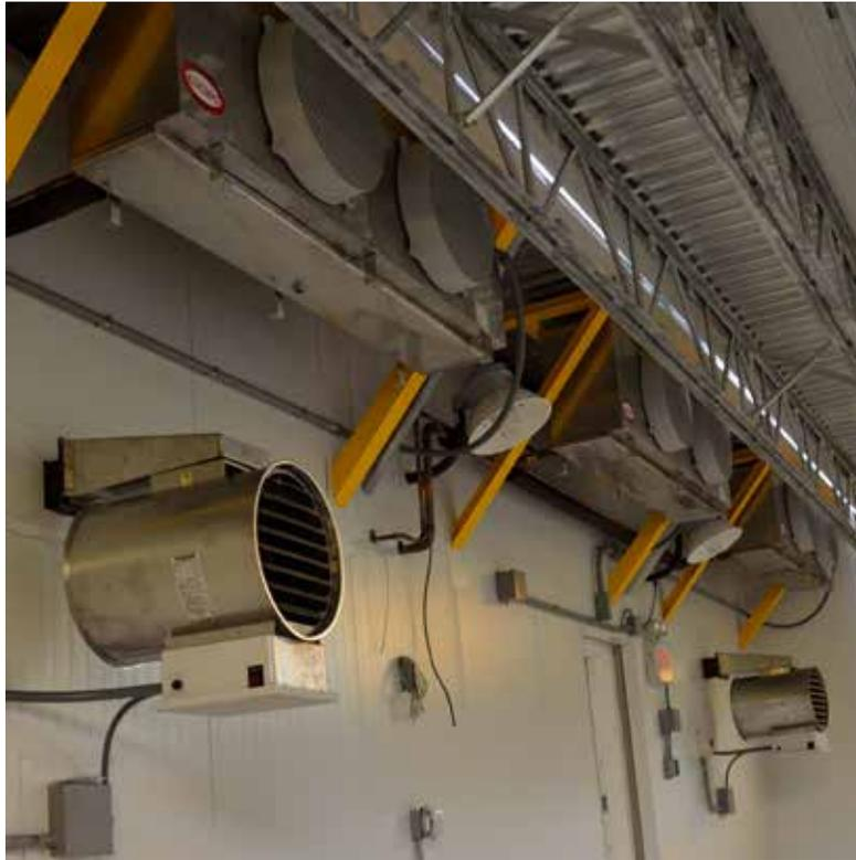
*Figure 31. HVAC Evaporators as Mounted in the Lower Environmental Enclosure. Heaters Also Shown.*
