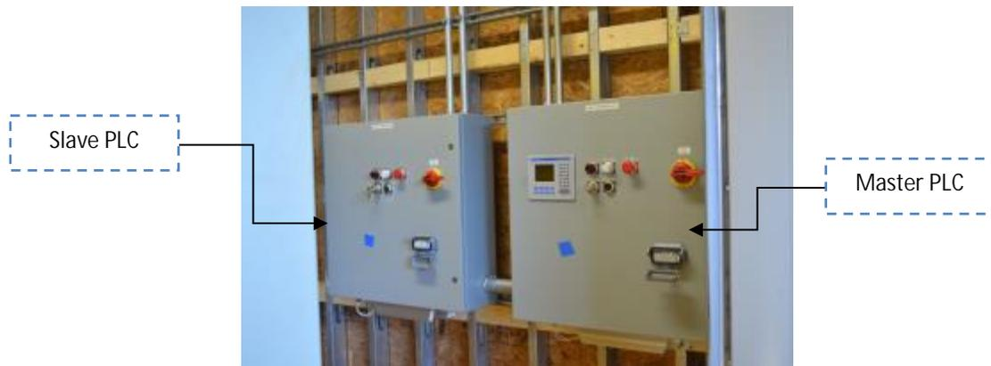
*Figure 7. Rail Cart Control System*
