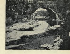
after the first money had been raised. Six years later the waterway was opened to traffic between Newark and Phillipsburg. Hand labor was the backbone of the construction job. Concrete, as used today, was unknown. All masonry had to be of stone construction, held together by lime mortar. There were no compressed-air drills or dynamite, no steam shovels or motor trucks, no iron girders or "I" beams. A working day was from sunrise to sunset. The wages were 90 cents a day or even less.
